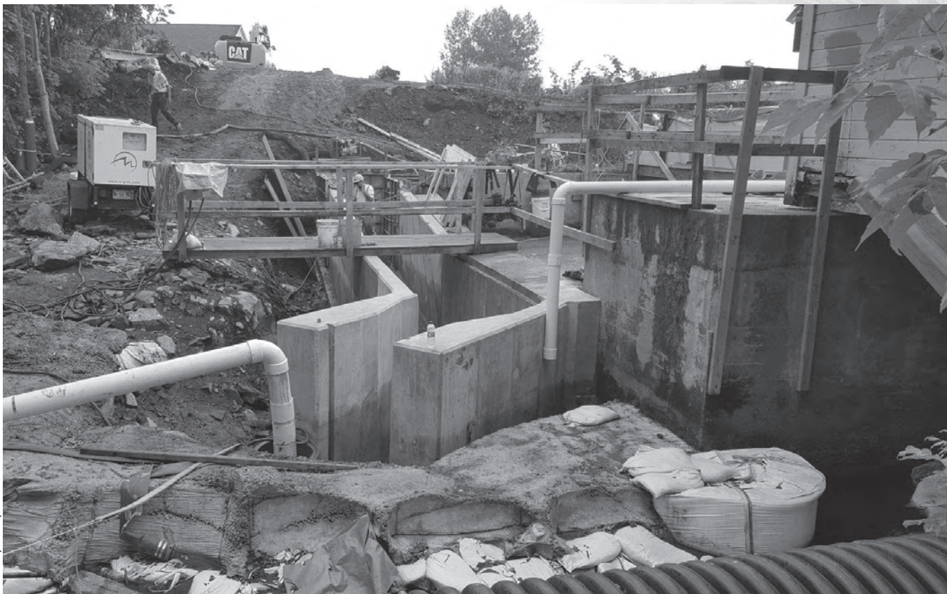
Construction of fishway at Outlet Stream Dam
