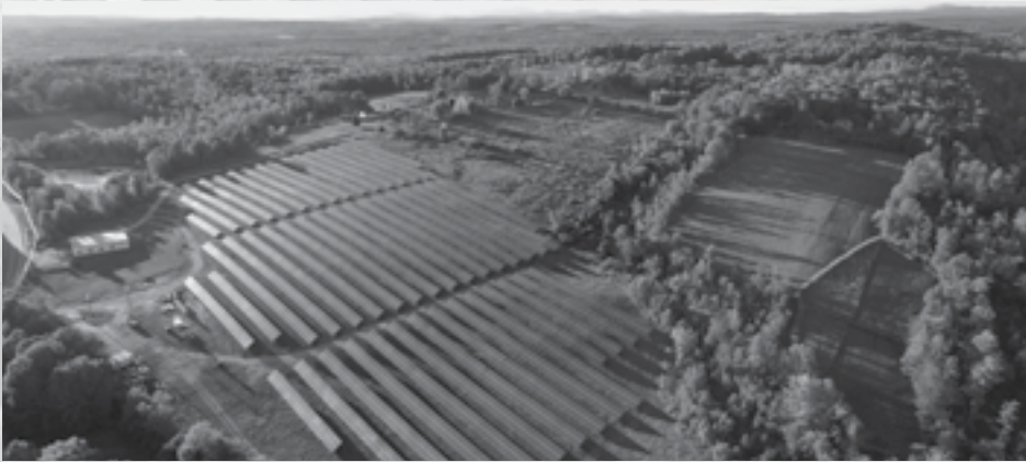
Solar Array in Skowhegan that is generating renewable energy for multiple municipalities, including Vassalboro.
