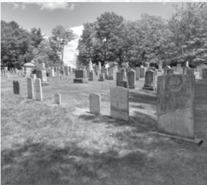
Before and After photos of stone repairwork contributed by Jody Kundreskas.
