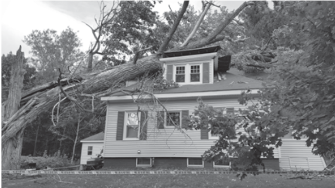
Fallen tree on house on Priest Hill Road
