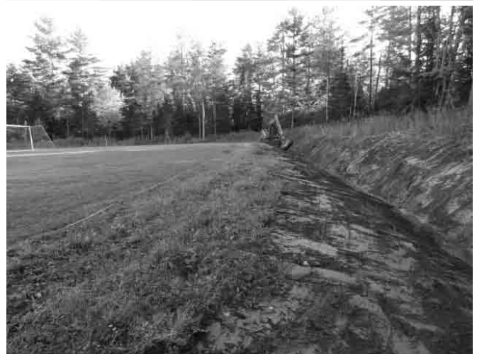
Drainage improvement project at the rec fields.
