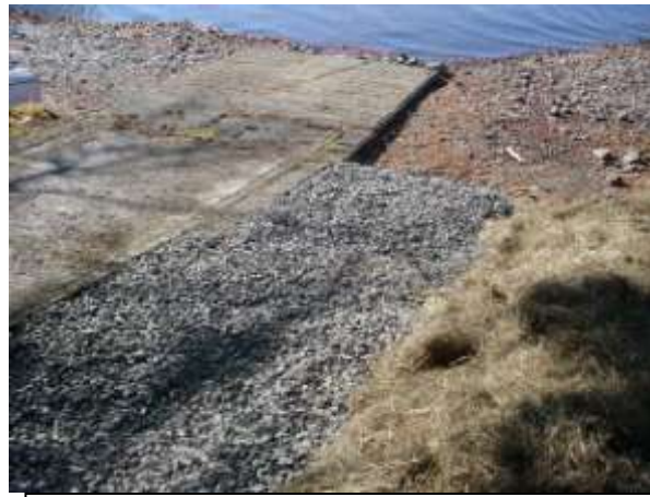
Boat ramp with infiltration trench installed #2 & #12
